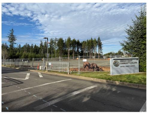
Site stabilization includes wood chip placement to mitigate erosion during wet weather.
